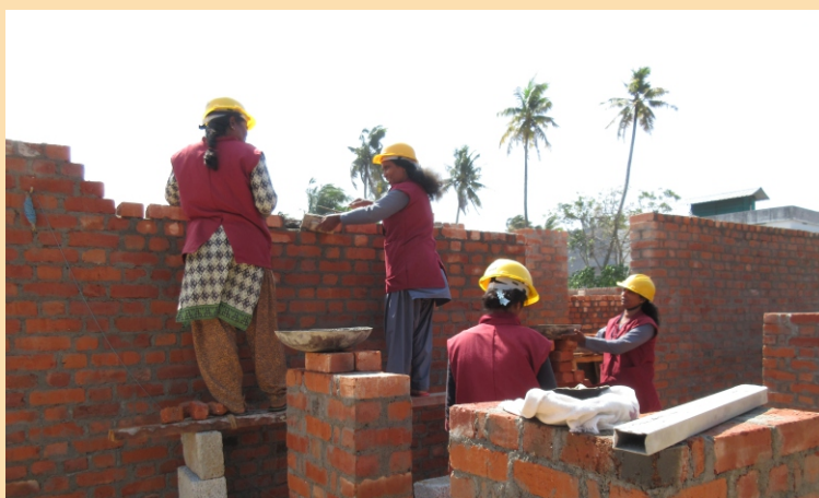
Women Construction Group under Kudumbashree Mission
